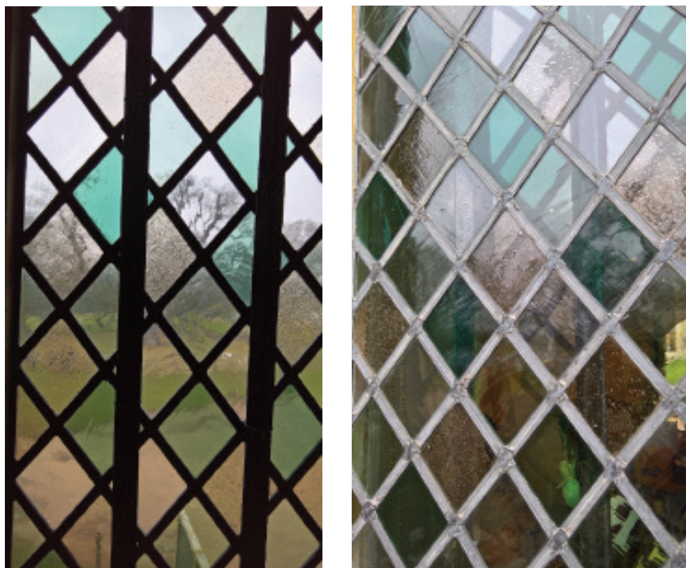
Fig. 5 Mauve and green-tinged leaded glass in situ at Knole; a) internal view, b) external. (Photo by S. Draper.)
