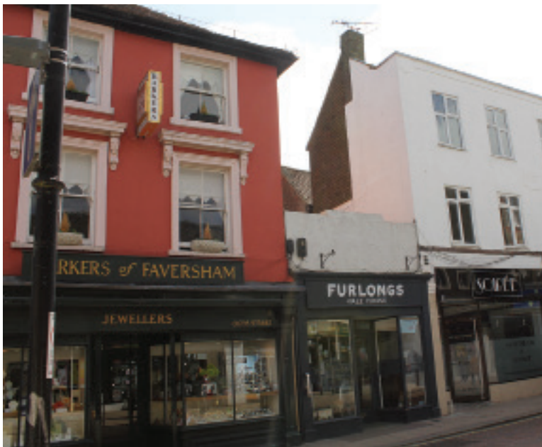
Fig. 7 Frontage of Furlongs in Preston Street in 2017. The white building to the right is the surviving two-thirds of the original No. 6.
