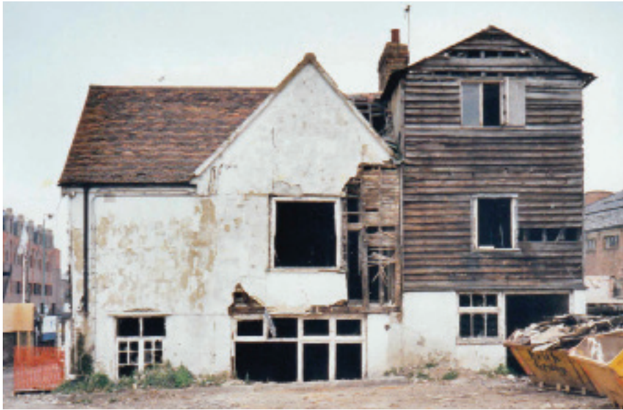
Exterior from the south showing the Phase-2 main range with added ranges to left and right.
