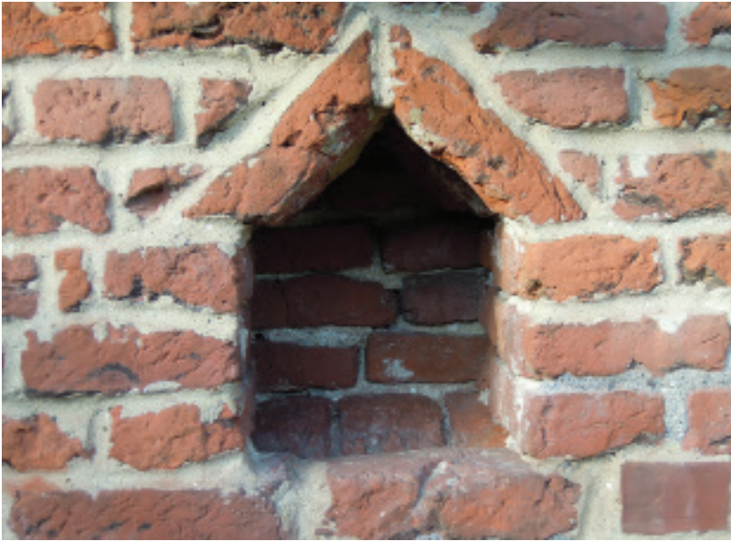
Fig. 1 The bee bole structure at Old St Albans Court, Nonington.
