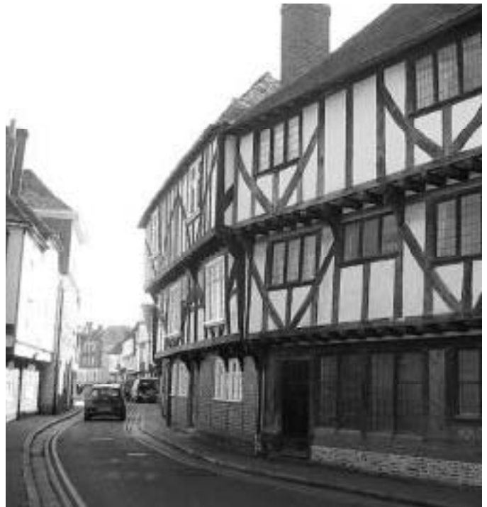
ABOVE: Strand Street house in Sandwich dated by dendrochronology to 1334.
