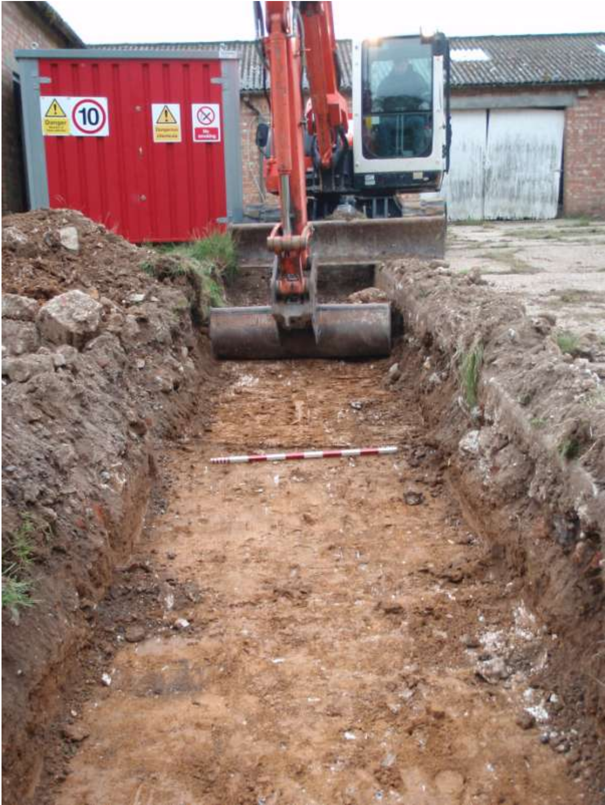
Plate 4 – Trench 2 with additional reduction (looking ESE), 1m scale.
