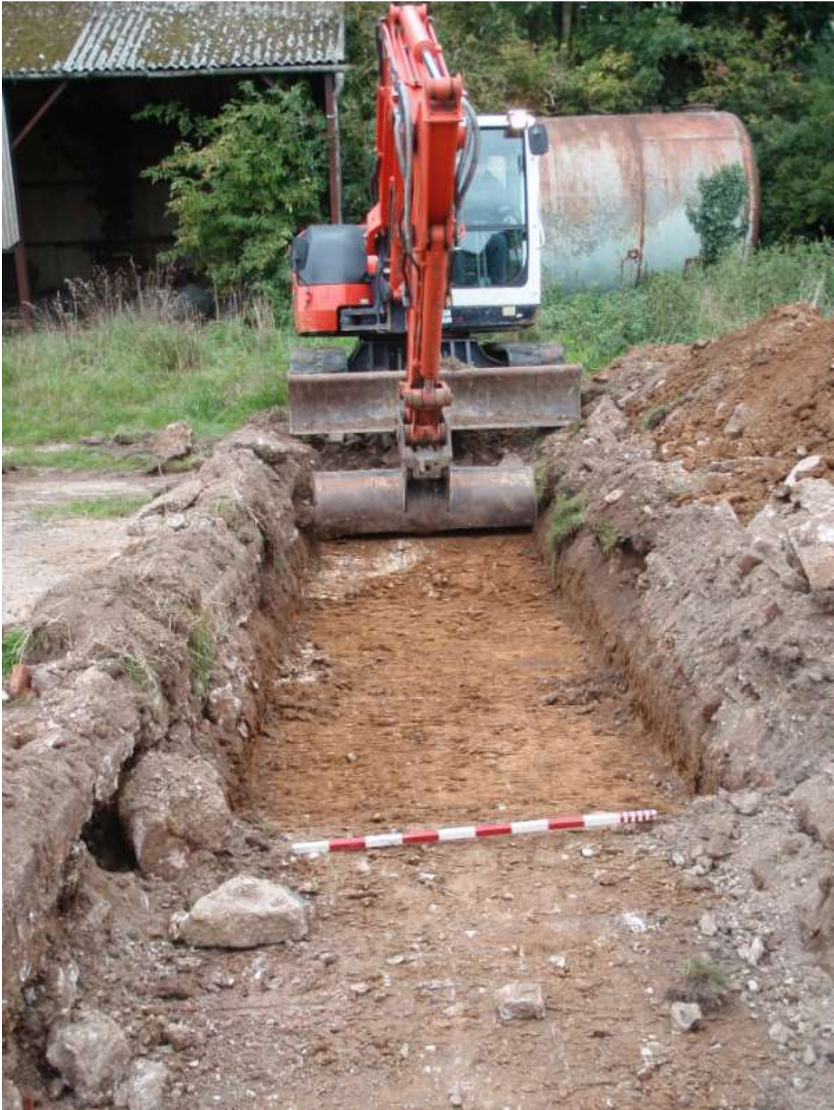
Plate 3 – Trench 2 with additional reduction (looking WNW) 1m scale.
