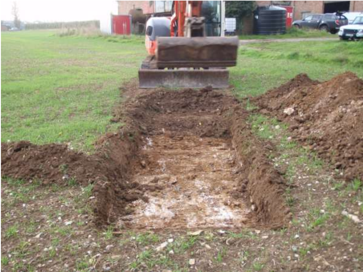
Plate 1 – Trench 1 under excavation (looking SSE)
