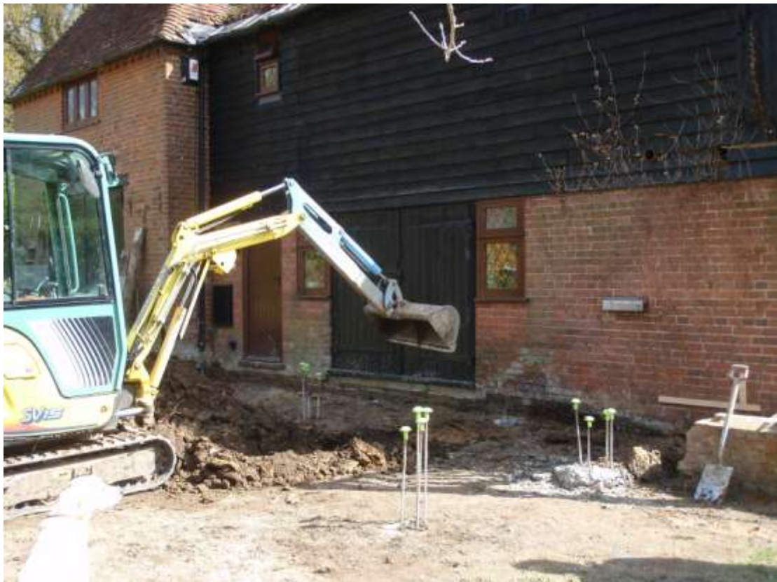
Plate 3. View of topsoil strip (looking east)
