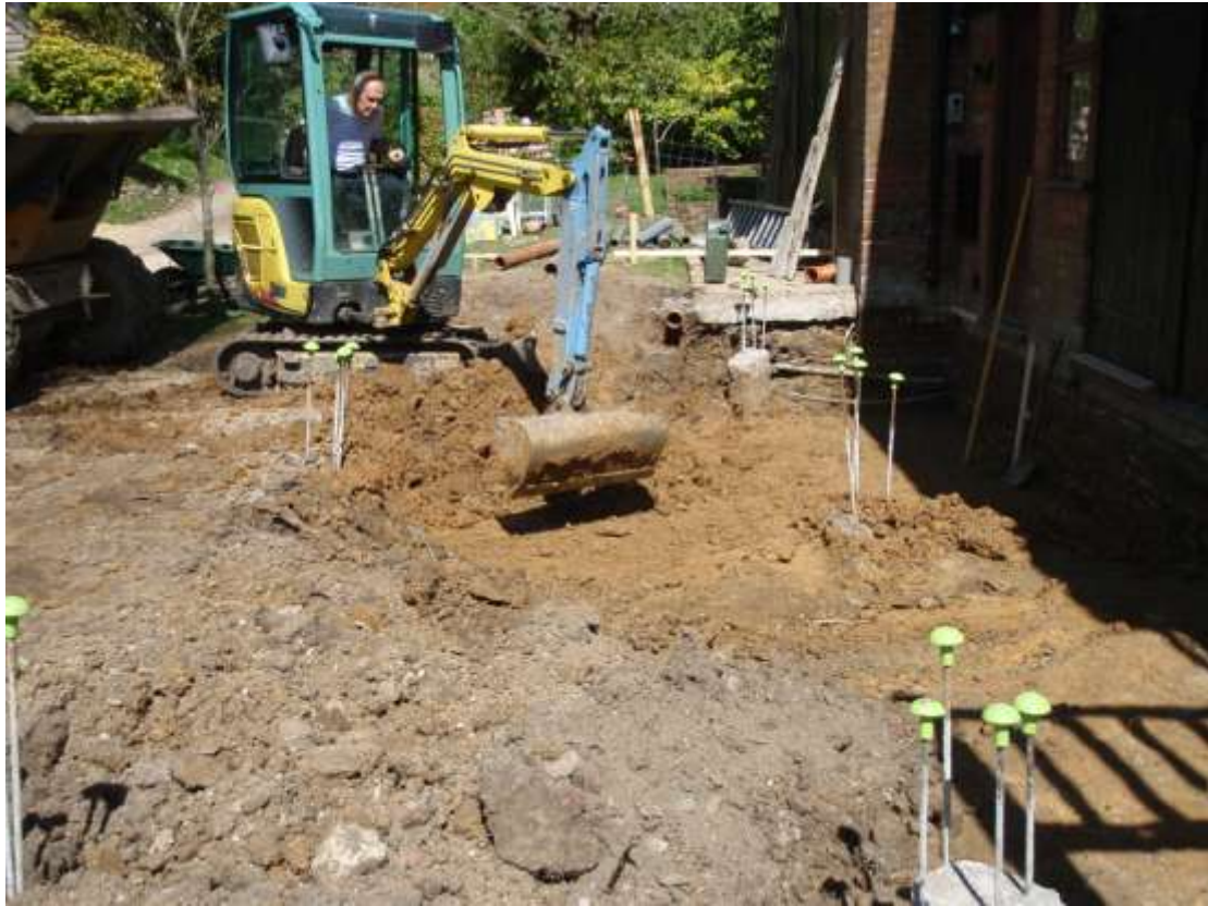
Plate 4. View of ground reduction
